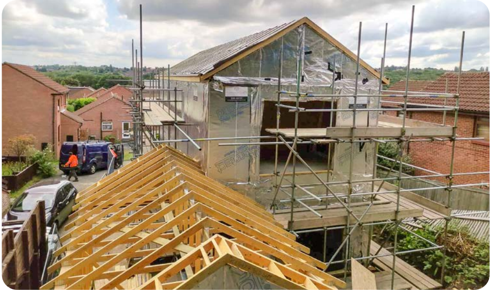
A new self-build home under construction
