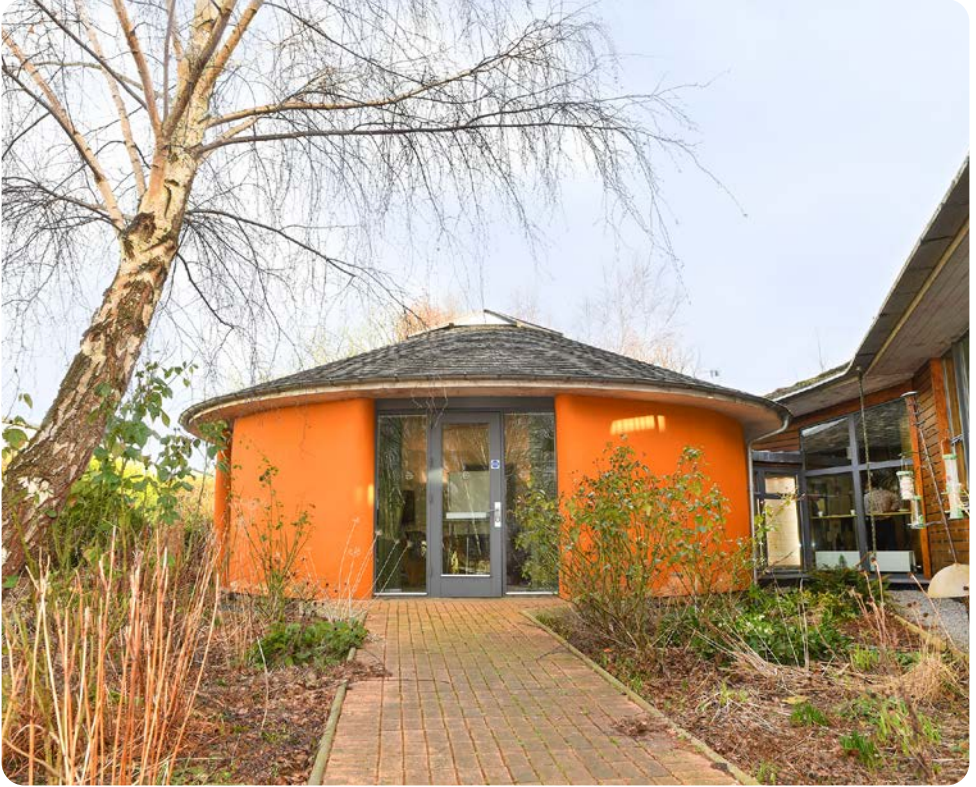
Ecology's straw-bale construction boardroom at our head office in Silsden, West Yorkshire
