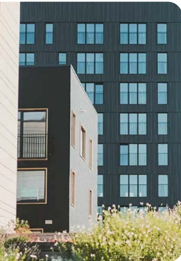
Leeds Community Homes project on the banks of the River Aire
