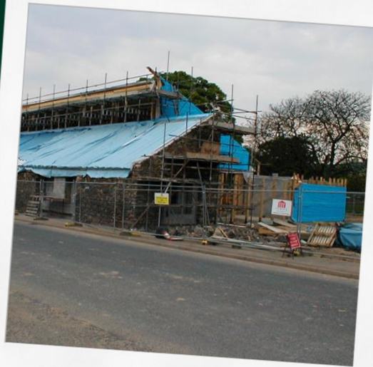
Silsden HQ under construction
